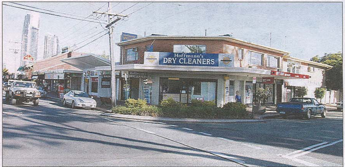
64 Thomas Drive . . . the refurbishment will include interior and exterior changes
