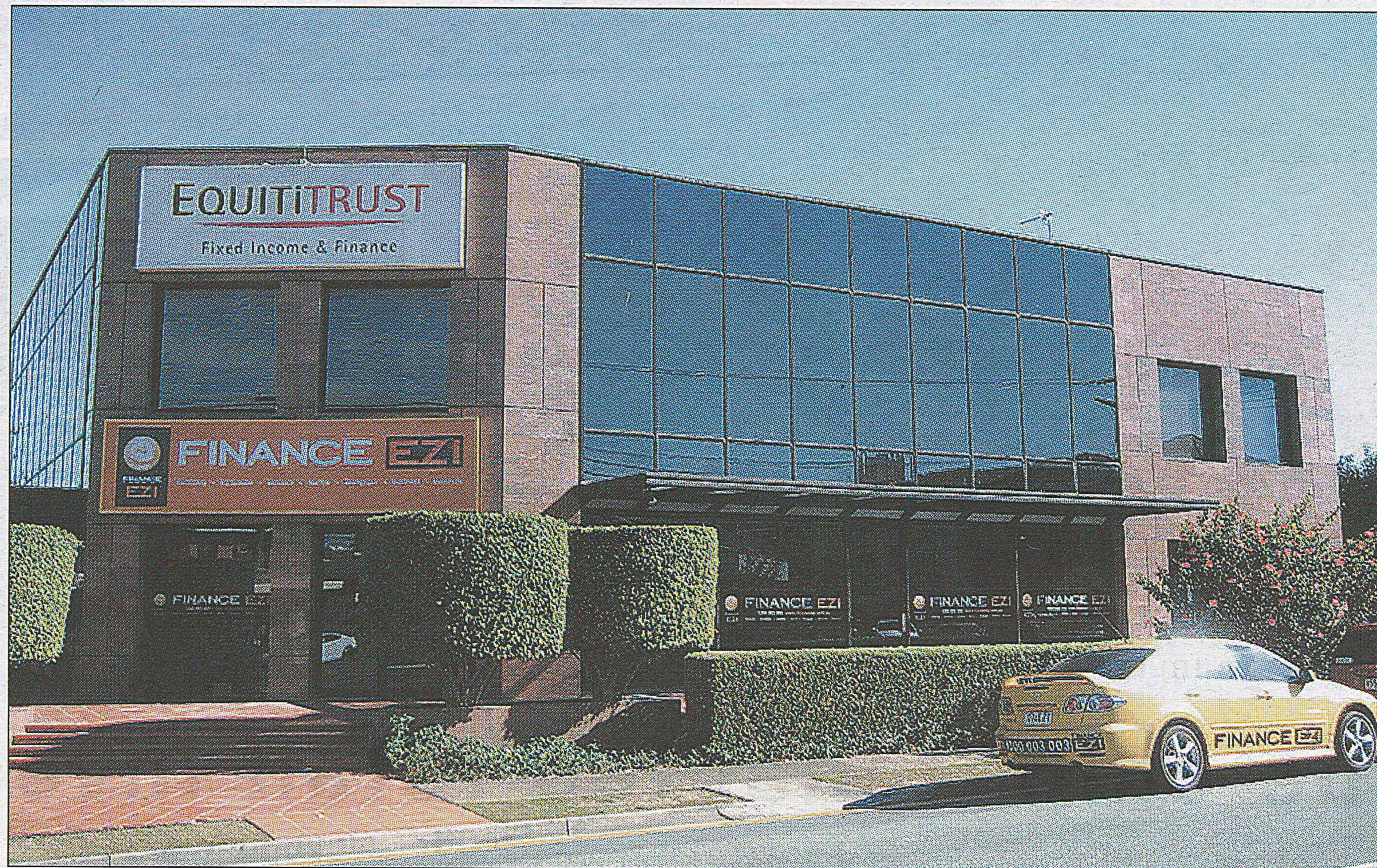
Finance Ezi's new home, a freestanding office building on Thomas Drive, Chevron Island
